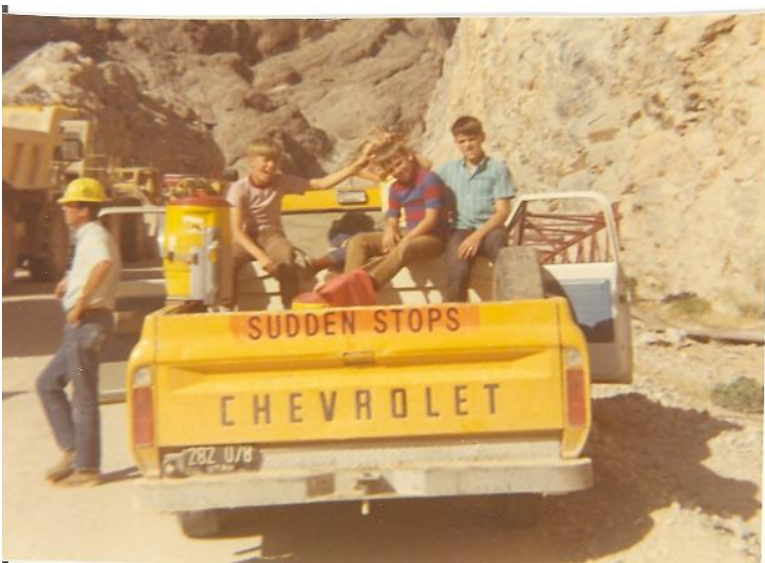
Note the 50 ton rock truck to the left of the photo
