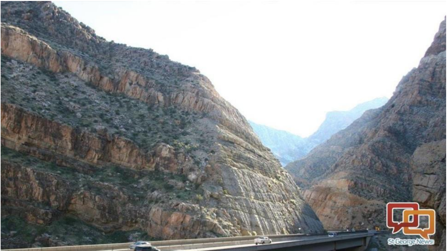
PHOTO OF BRIDGE SIX, looking South downstream.
